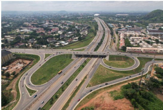
WUYE FLYOVER BRIDGE, ABUJA
