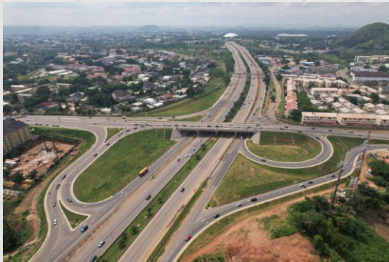
WUYE FLYOVER BRIDGE, ABUJA
